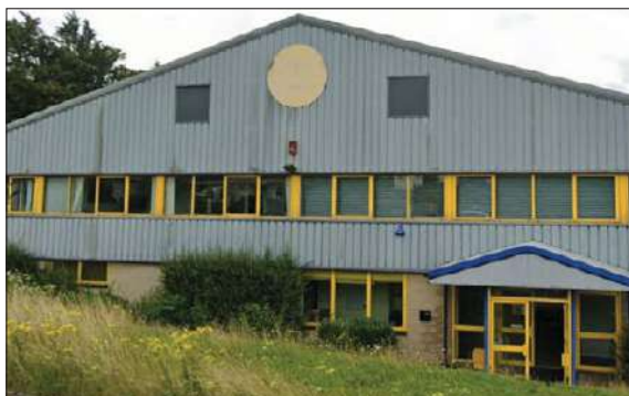
The indoor tennis centre opened on November 1, 1993
